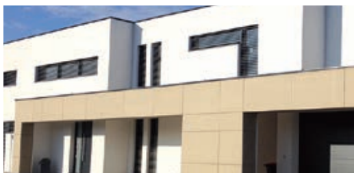
Facade insulating boards with DKF TOP coating.
